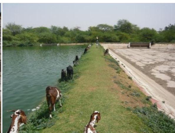
Figure 6: Maturation ponds: left side operational, right side not functional
