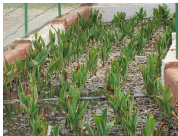
Figure 35: Treatment unit planted with canna indica
