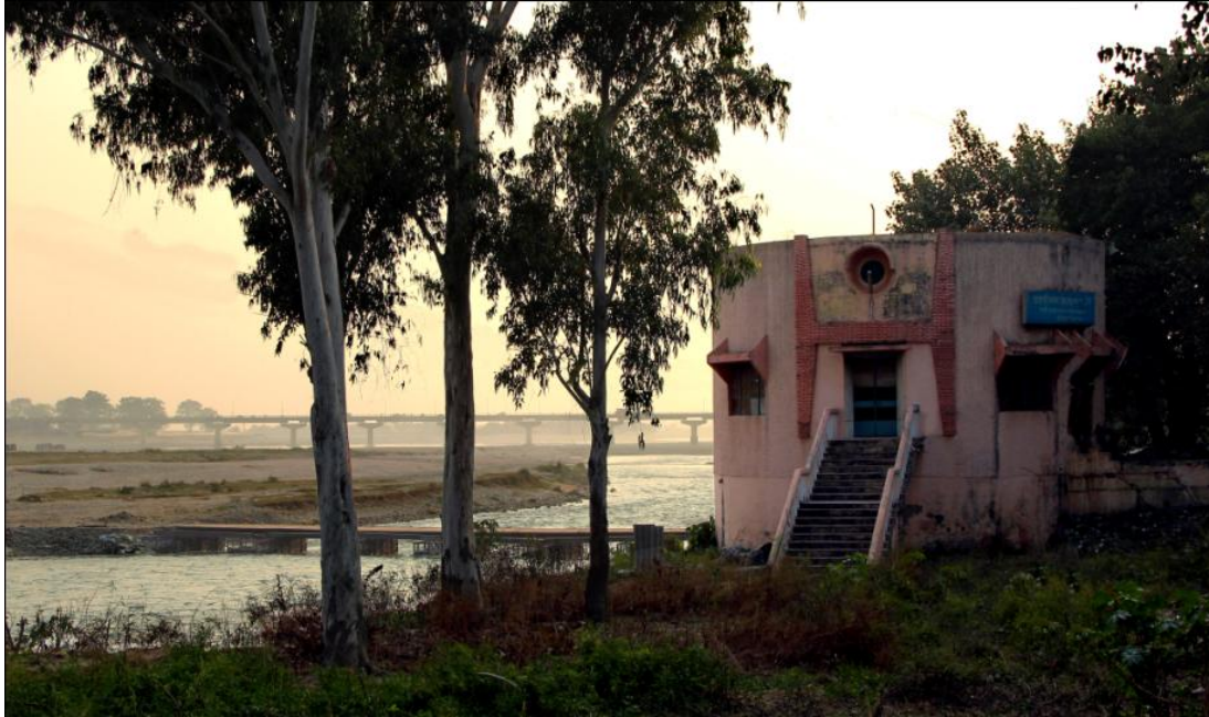
Figure 63: Example of a large-diameter RBF caisson well adjacent to the Ganga River in Haridwar (Photo: L. Rossoff, HTWD, 2011)
