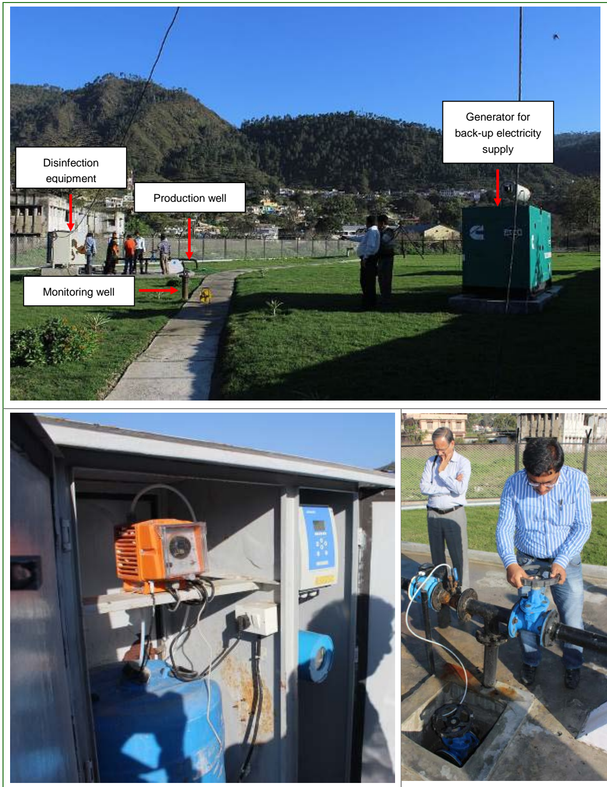
Figure 3 Production well at RBF site in Srinagar (top) by the Alaknanda River in Uttarakhand operated by UJS, the disinfection dosage pump (bottom left) and the disinfectant supply pipe (bottom right) to the drinking water distribution pipe from the well (Photos: HTWD, 2013; Installation of disinfection system: courtesy SME Simplex Control Equipments)
