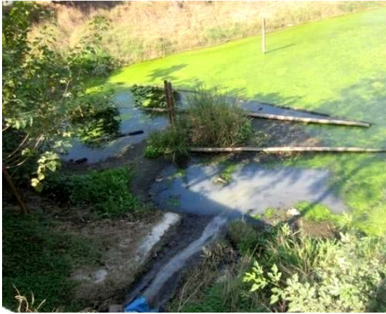
(A) Pre-treated discharge of influent into duckweed pond at Sandhuan, Roop Nagar, Punjab
