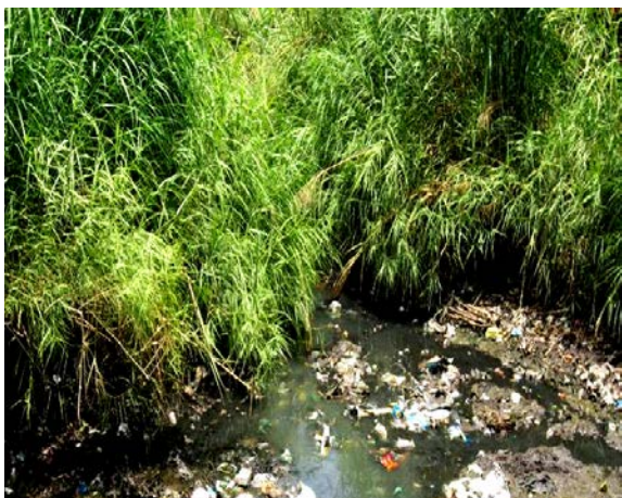
(C) Absence of pre-treatment unit resulted in clogging of CW bed
