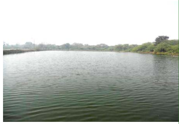
Picture 2: WSP, Masani, Mathura, Uttar Pradesh, India
