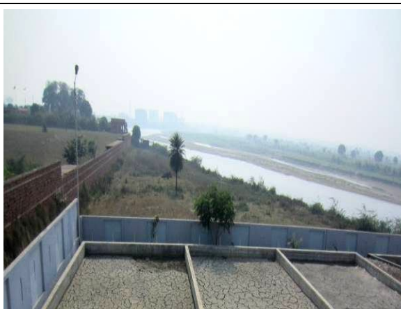
Picture 5.12: Treated wastewater discharge into River
