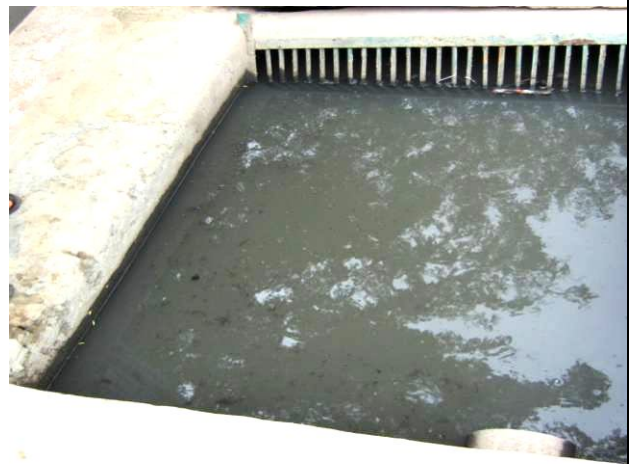
(A) Primary Treatment Unit(Grit Chamber)
