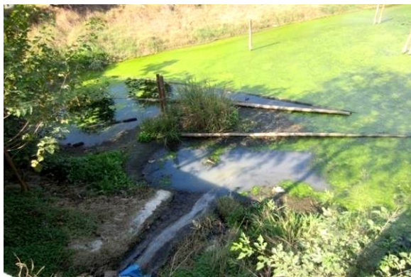
Picture 3.13 : Absence of primary treatment unit at site code; India_PB_7_DP
