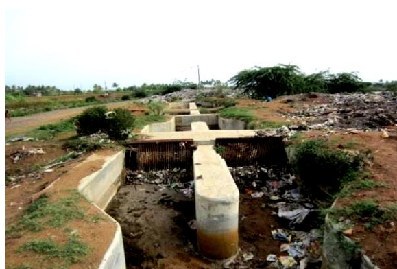
Picture 3.10 : Status of lack of cleaning to primary treatment unit at site code; India_MH_3_WSP
