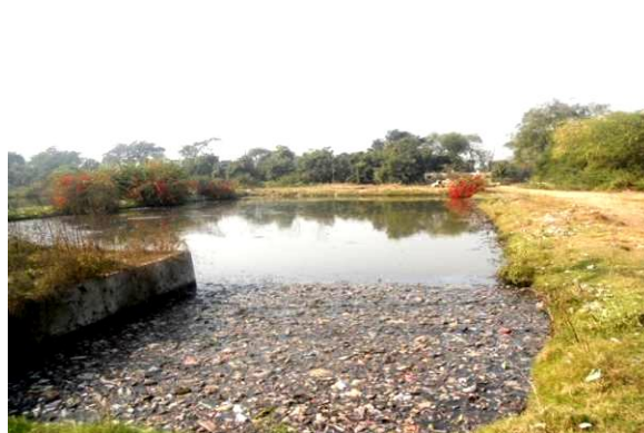
Picture 3.8 : Effects of non-functioning of primary treatment unit in at site code; India_UP_7_WSP
