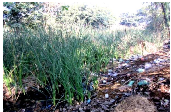
Picture 3.6: Status of lack of cleaning of CW bed at site code; India_PB_6_CW
