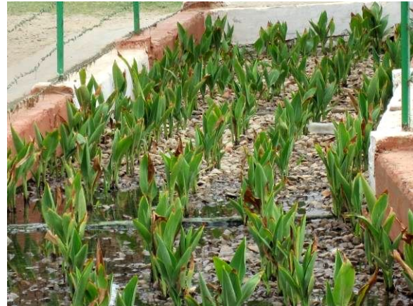
Picture 5.6: Constructed wetland bed for wastewater treatment
