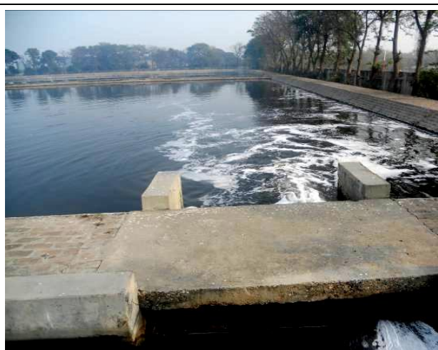
(C) Inlet of Polishing Pond
