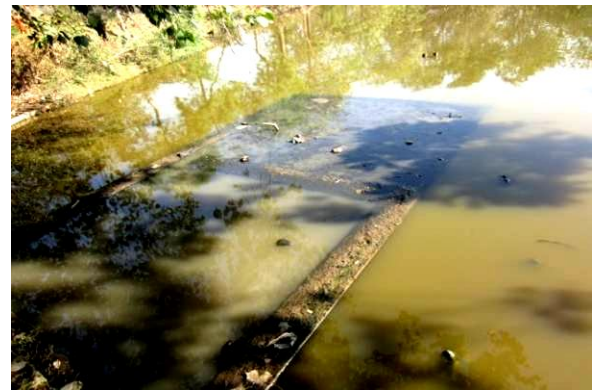
Picture 3.12 : Status of submerged primary treatment unit at site code; India_PB_8_DP
