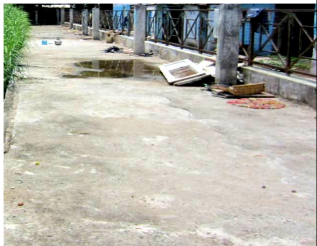
(A) Primary Treatment Unit
