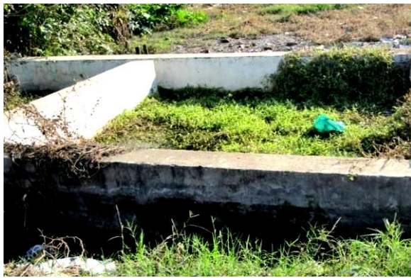
Picture 3.11 : Status of lack of cleaning to primary treatment unit at site code; India_PB_10_DP
