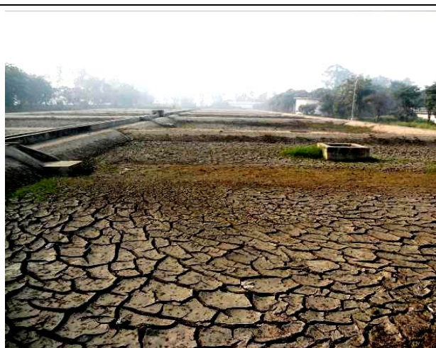
(E) Sludge Drying Beds
