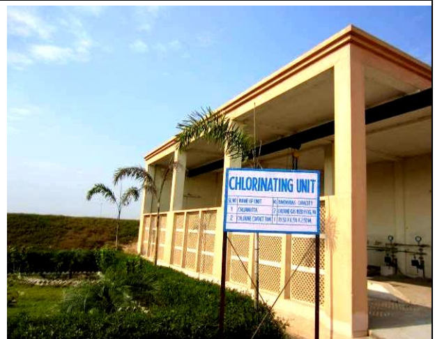
(E) Chlorination Unit
