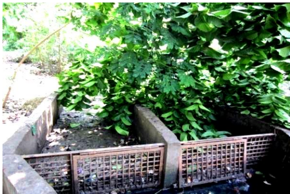
Picture 3.3: Status of irregular cleaning of primary treatment unit at site code; India_MP_6_CW
