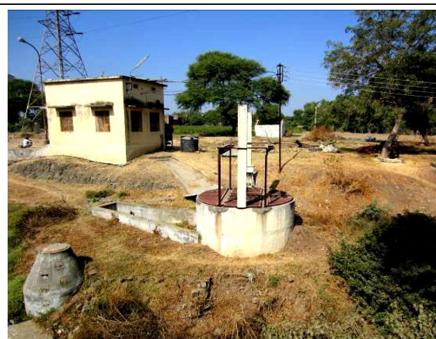
(B) Pump House
