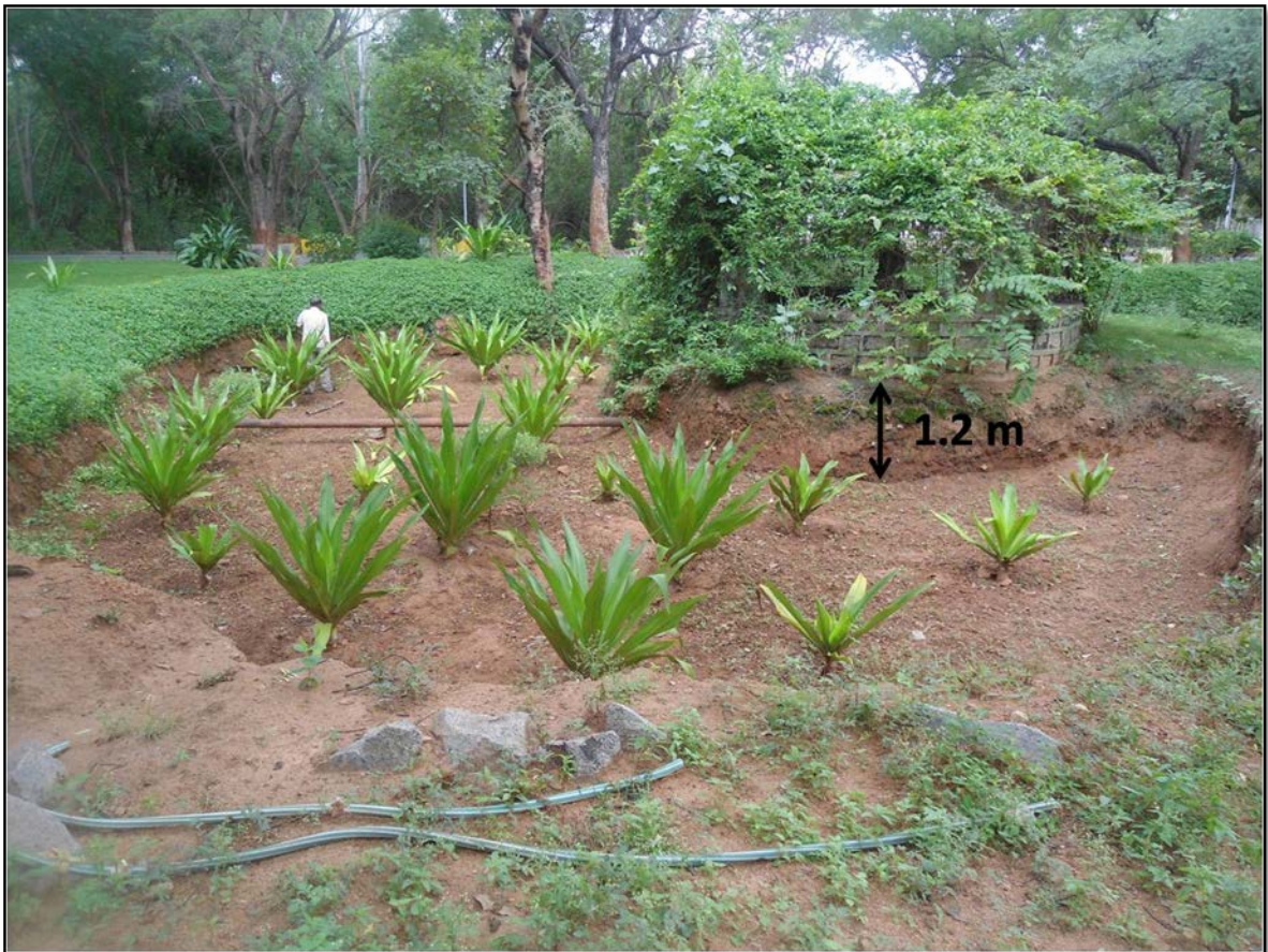
Figure 5-7: Rain gardens constructed in the upstream side of the NGRI Campus after the results of the time lapse experiment. The monitoring bore well BW3 is within this site, but outside the rain garden
