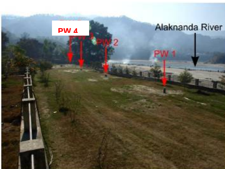
Figure 4-2 View of four additional production wells installed in August 2011
