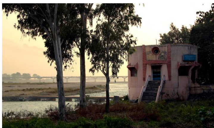
Figure 2-2 Example of large-diameter RBF well adjacent to Ganga River, Haridwar (Photo: L. Rossoff, HTWD, 2011)
