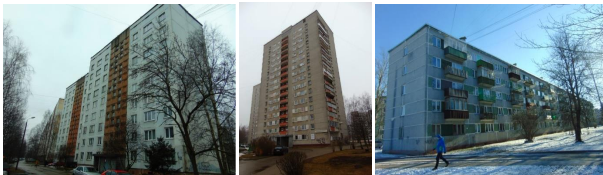
Figure 69. Examples of multifamily buildings built in time period from 1946 to 1993
