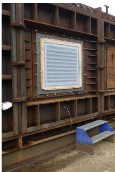
Fig 6. Plastic sheet covering the grille
