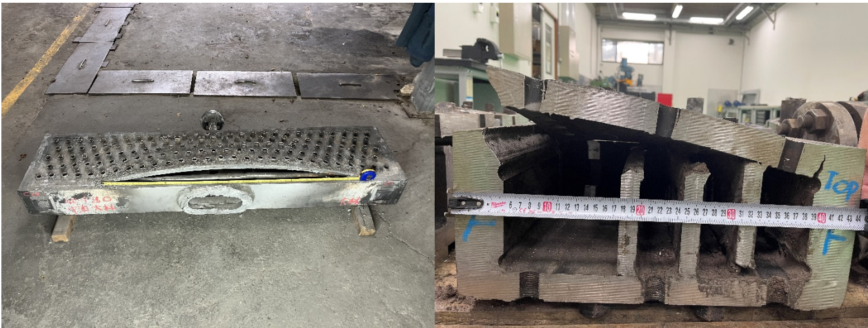
Fig. 5. Photo of cut-out of E-3004A outlet side header box
