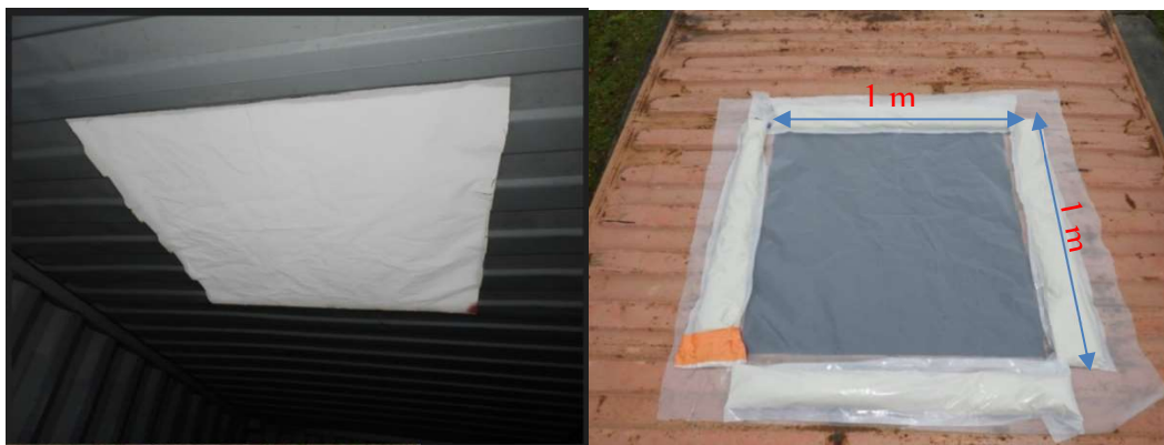
Fig. 2. Inner and outer views of the vent on the container roof.
