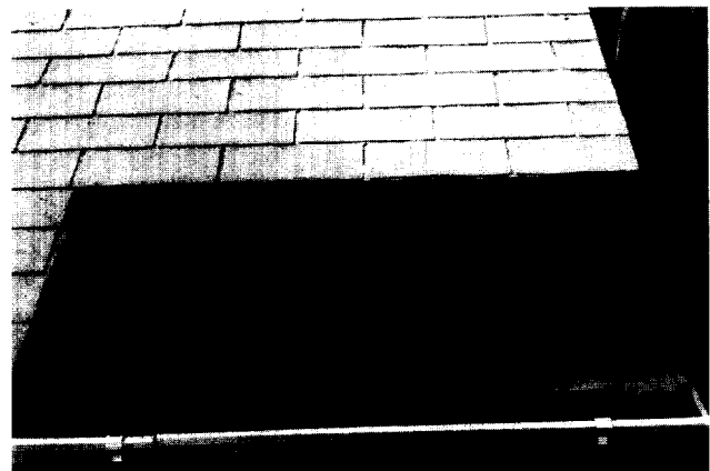
Fig. 2. Photograph showing an asphalt shingle roof that was partially coated with a high albedo coating. The uncoated (dark colored) shingles have contracted and cracked but the shingles have not. Courtesy of Bill Kim, Rohm and Haas Company.
