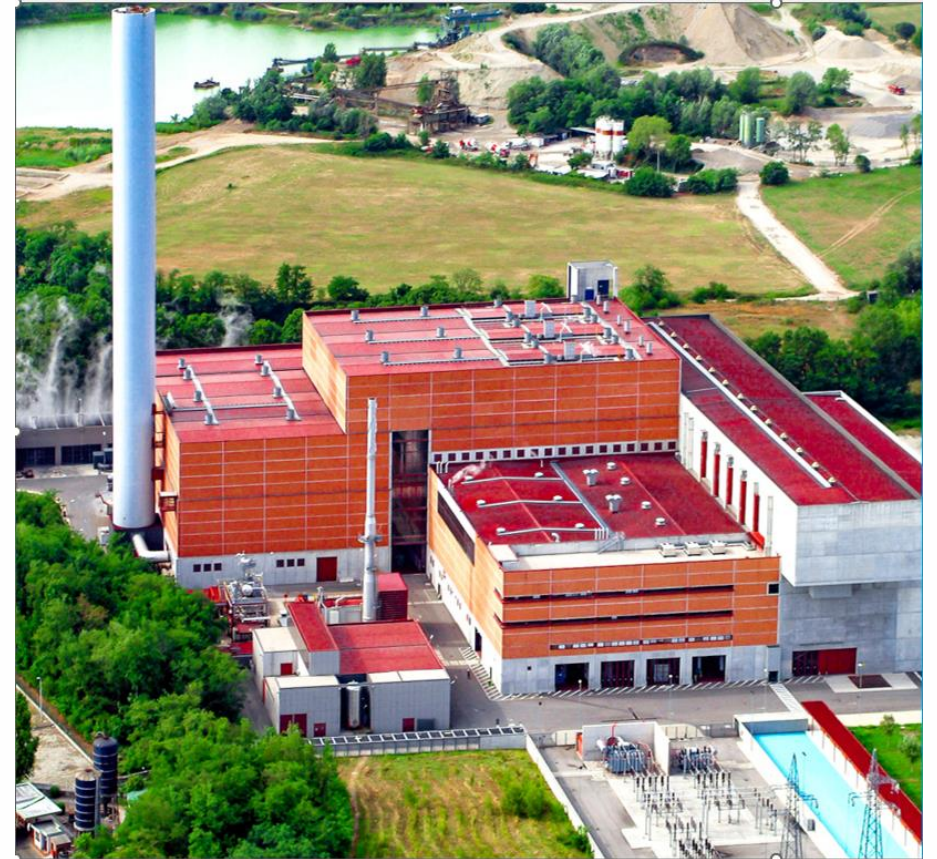
WtE Plant Milan – CaL Pilot Plant Installation Site
