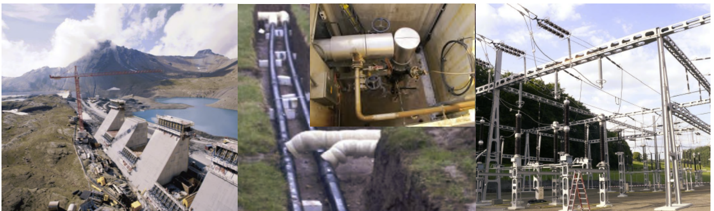
Hydro dam Mutsee, Glarner Alps
