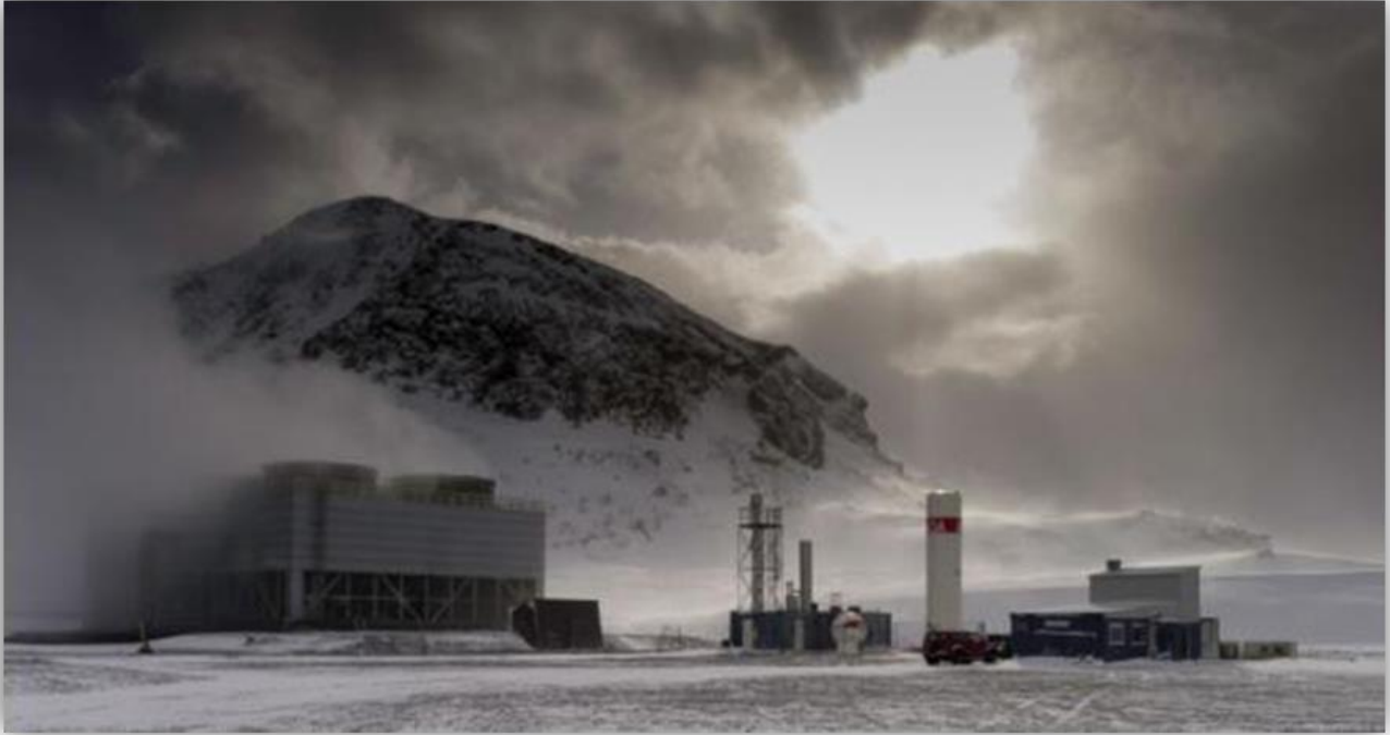
Figure 14 Gas laboratory at Hellisheiði Power Plant, (photo: Orkuveita Reykjavíkur)
