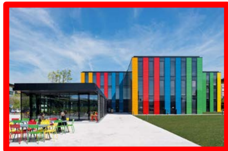
Central services building 2013
