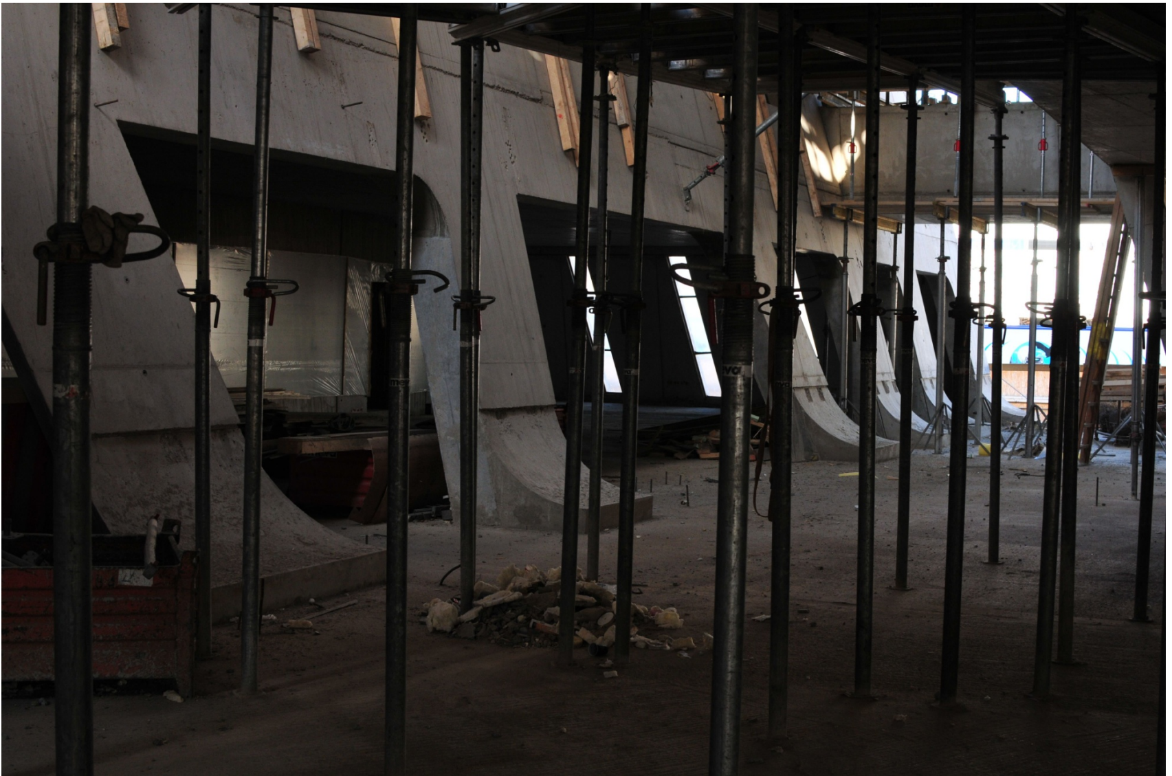
Shell construction of canyon wall May 2012
