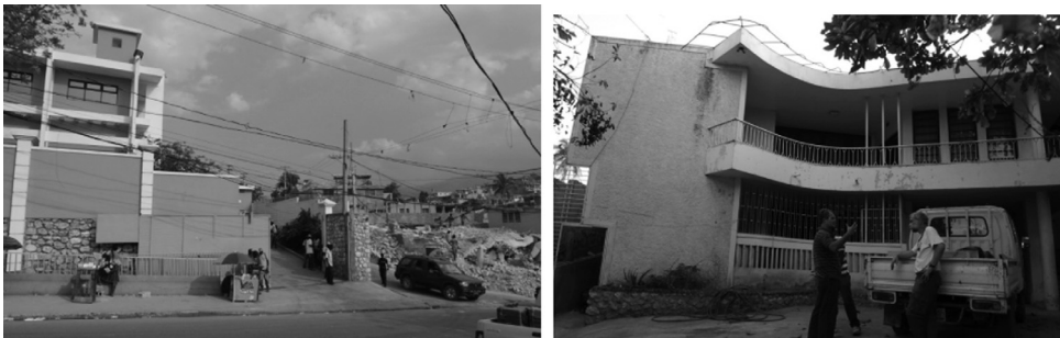
Figure 9. (a) A good-quality commercial structure in which MMI V-VI is estimated based on an eyewitness interview; (b) a private home, masonry C construction, for which MMI VI is estimated. The structures on both sides of the structure shown in 8a collapsed catastrophically, as did a school building adjacent to the house shown in 8b.
