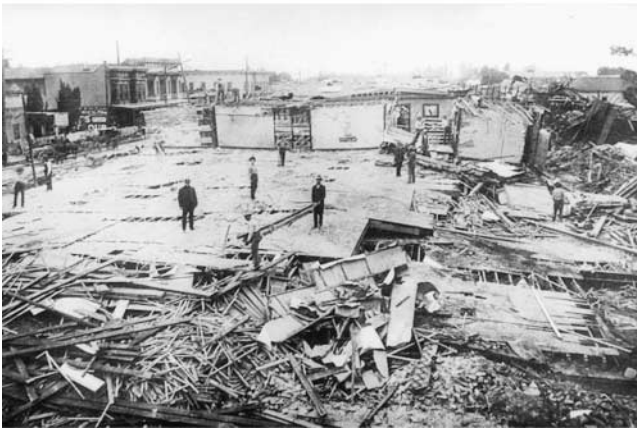
Figure 1. Photos showing damage in downtown Santa Rosa after the 1906 earthquake (from the Karl V. Steinbrugge Collection, Earthquake Engineering Research Center, University of California, Berkeley).
