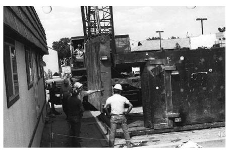
Figure 4. Shielded room construction at the IVRRF.
