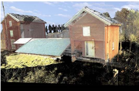
General views from the point cloud
