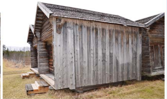
General views of the building
