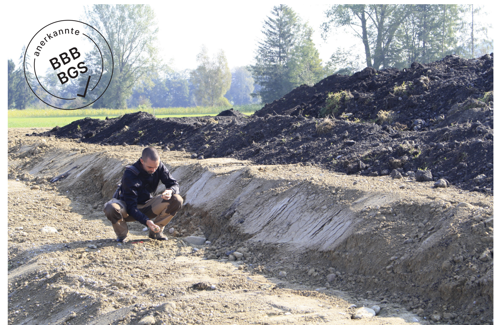
FIGURE 4: Large construction sites require a soil protection advisor to assure for appropriate soil handling on site. The SSSS is critically involved in the certification and quality assurance of the SPAs.
