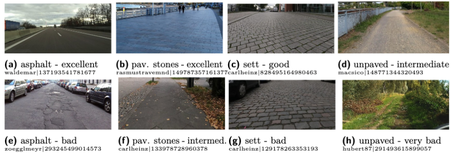
Figure 1: Example images of different surface types and qualities, with Mapillary contributor names and image IDs.
