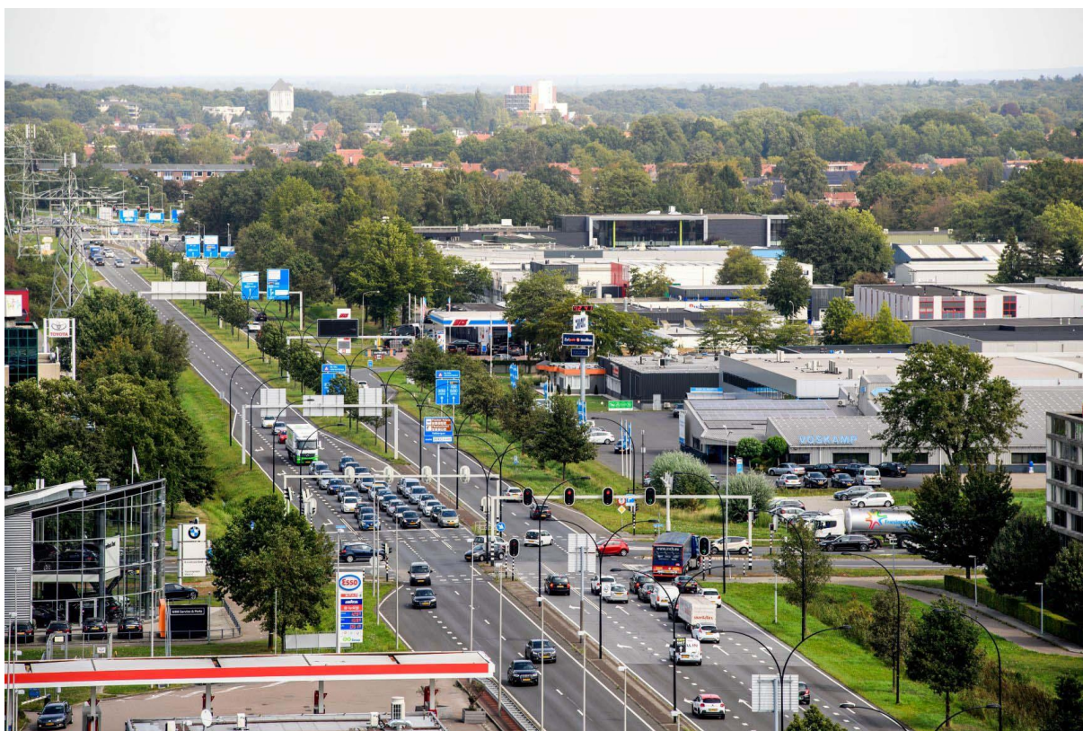
Figure 2 – One of the traffic signal intersections on an Almelo access road
