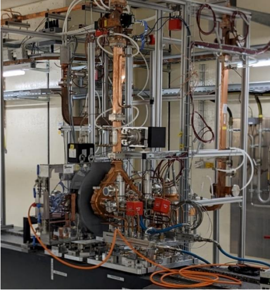
Fig. 3 High-power test stand realised and operational.
