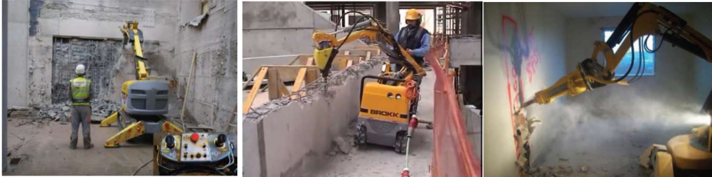
Figure 11 – Brokk demolition machine used in [31]
