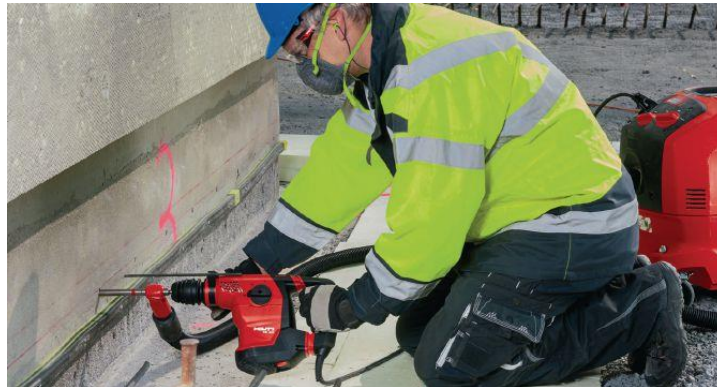
Figure 2: Concrete drilling
