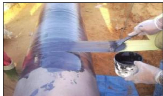
Fig. 6 Wrapping process of Kevlar tape repair system
