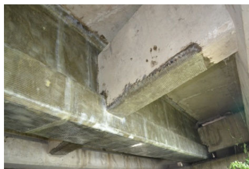
Fig. 1 Strengthening of Bridge Girder
