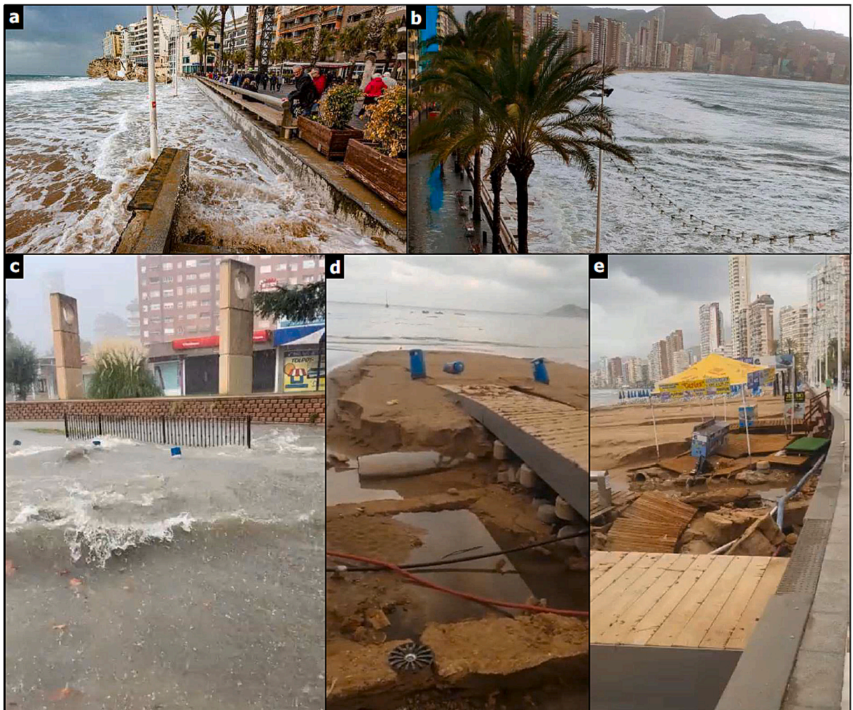
Fig. 2. (a-b) State of Levante Beach during ‘Gloria’ storm in January 2020 in which the waves hit the promenade, (c) Floods in the centre of Benidorm on 11 November 2022, (d-e) Damage caused to Levante Beach by the storm on 18 September 2022. Source: UA Climatology Laboratory.
