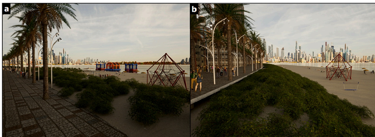
Fig. 9. (a) Urban dune at low points of the promenade, (b) Urban dune where the height of the promenade is sufficient to contain maritime flooding,
