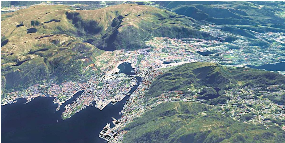
Fig. 1 The 3D map of the project domain in central Bergen. The domains include areas of required project application cases: Bergen Port; Tunnel entrances (Fjelltunnelen, Damsgårdtunnelen, Bytunnelen, Arnatunnelen); Major road conjunctions (Bystasjon, Danmarks plass, Puddefjordsbroen); Major parking houses; Major cultural objects (UNESCO Bryggen, Grieghallen) and shopping malls.
