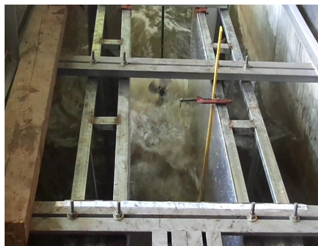
Fig. 6 Turbine placed at the tunnel end
