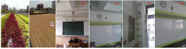
Fig. 4 The measured points in green roof and interior classroom
