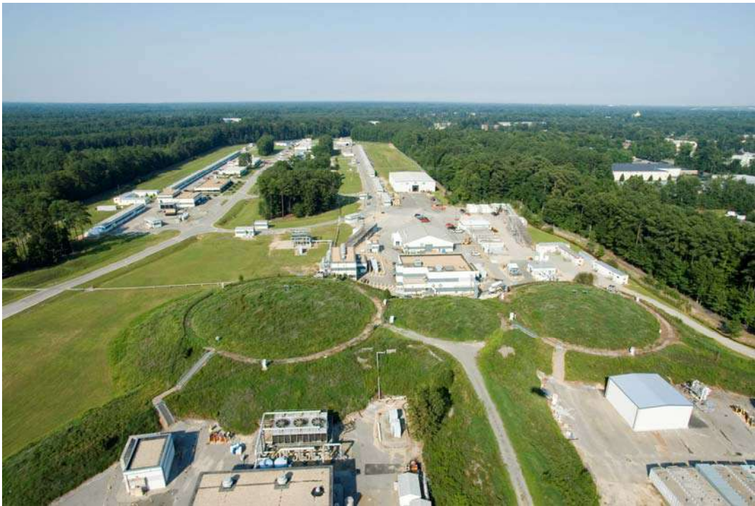
Aerial photo of the Jefferson Lab accelerator site
