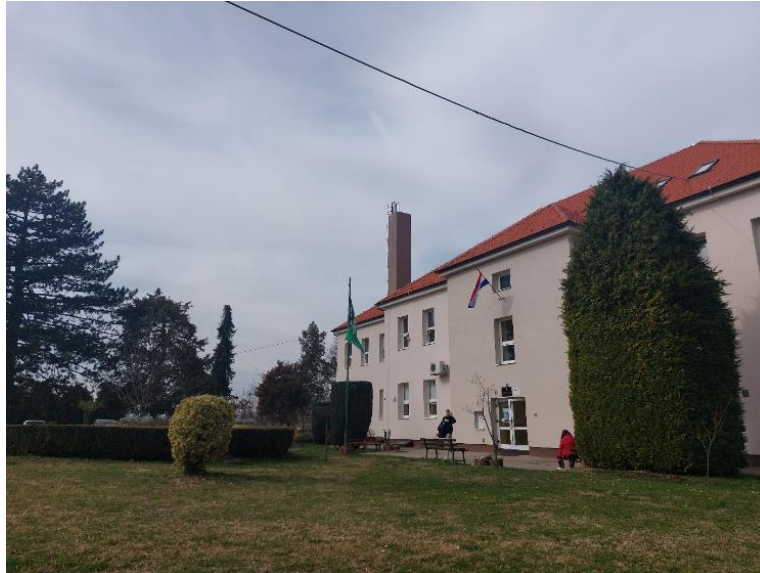
Upper-secondary school Ilok
