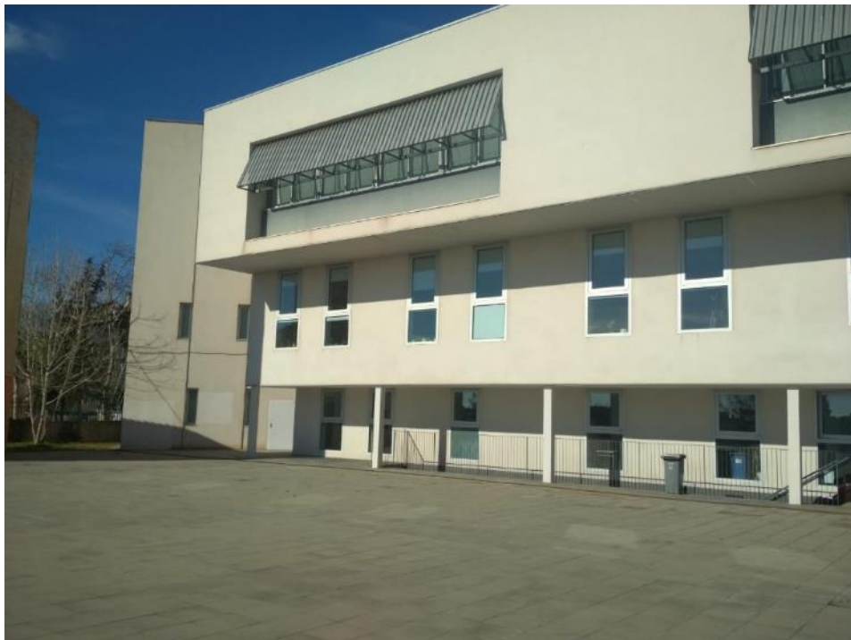
The main building of the school
