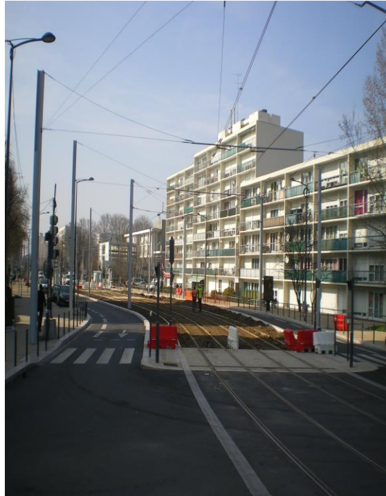
Local tramway under construction
