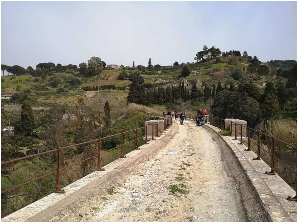
Figure 4: Old railway bridge between Calatafimi and Vita
