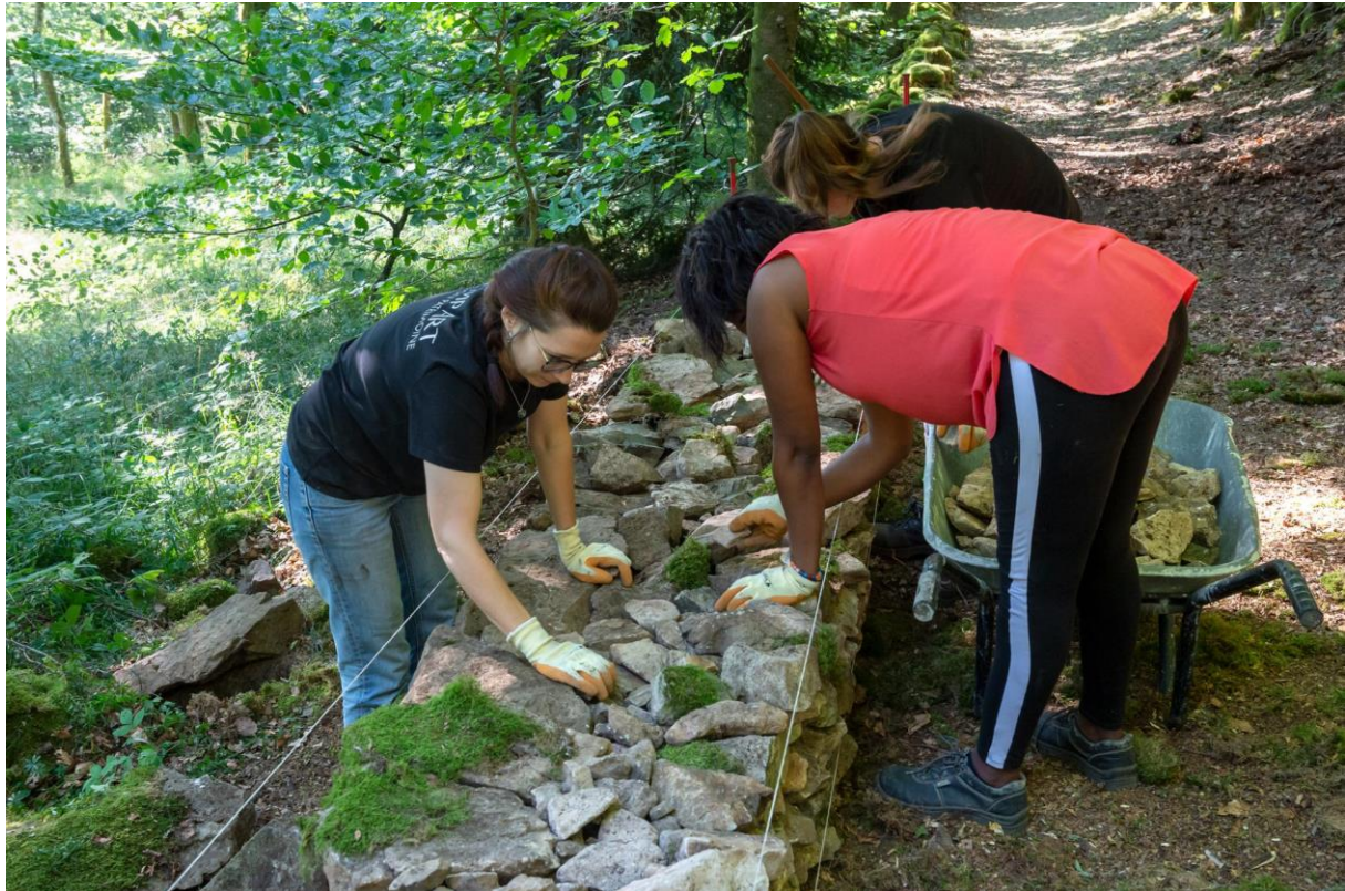
Figure 6: Workshop by the association Rempart on dry stonewall building 2023.
