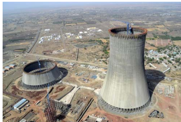
Fig. 1 Construction of Kalisindh thermal energy plant in Rajasthan, India
