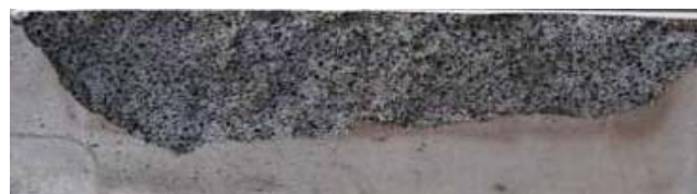
Fig. 4 State after testing – spalled concrete
