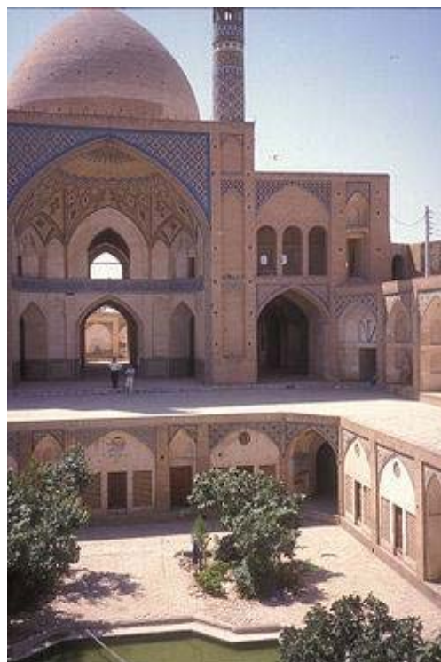
Fig. 13 Aqa Bozorg Mosque in Kashan (1778)
