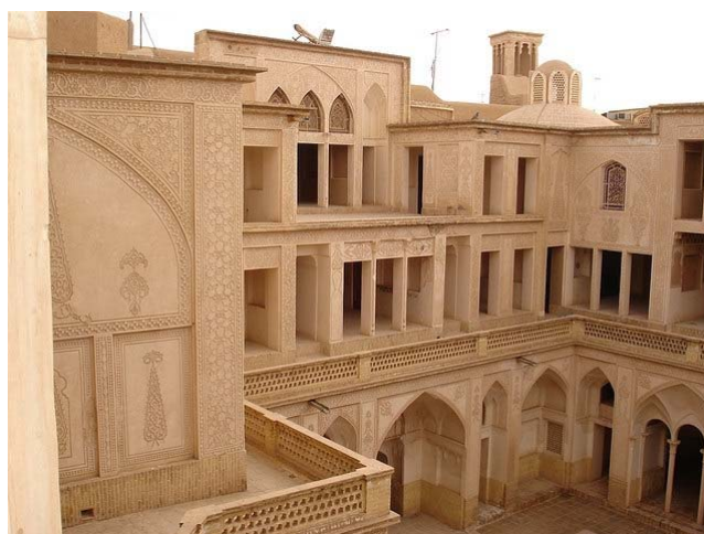
Fig. 10 Abbasian House, Kashan, two floors on top of basement
