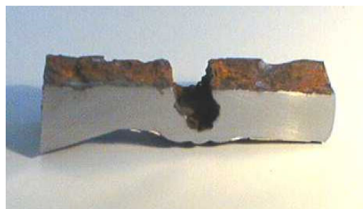
Fig. 1 Severe preferential weld corrosion in carbon steel pipeline carrying inhibited oil and gas [8]
