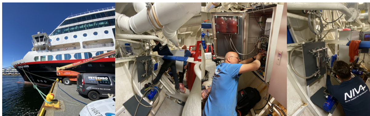
Figure 74: The installation of the microplastic sampling module in the pump room of the Hurtigruten M/S Trollfjord.
