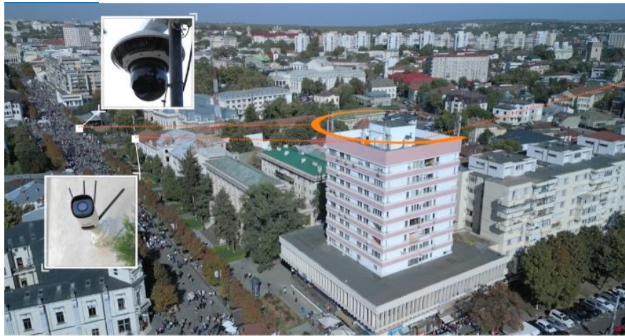
Figure 11. Camera's position on Stefan cel Mare Boulevard.
