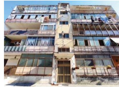
Figure 2: Detail view of the southern façade of the pilot building
