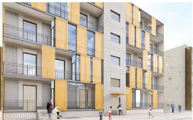
Fig. 9b: Sliding panels in perforated metal sheet on the south side
