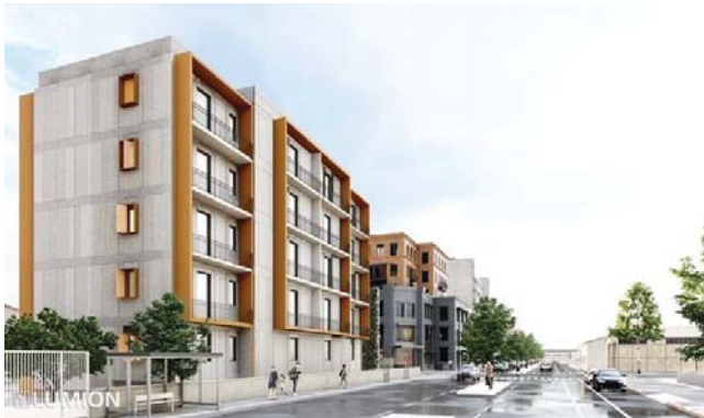
Fig. 8a: Coplanar ceramic tiles that are all bound together through a rigid substructure.
