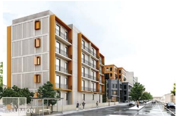
Fig. 8b: no-coplanar ceramic tiles that are all bound together through a rigid substructure. This expedient emphasizes the compositional rhythm of the e-SAFE panels and the geometry of the stringcourses.
