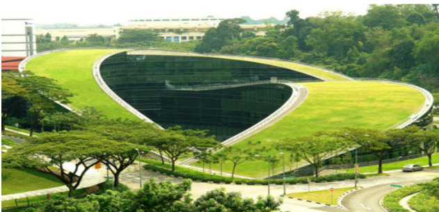
Fig. 4 Green roof on school of Art, Design and Media at Nanyang Technological University in Singapore
