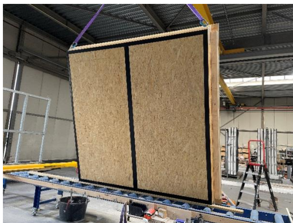
Figure 14: Waterproof finish of the back-wall test cabinet
