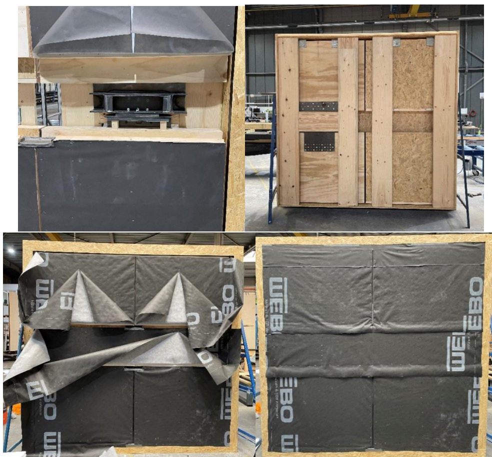
Figure 12: Placing the upper right element according to the e-CLT panel
