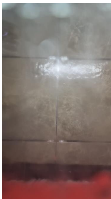
Figure 33: Façade element during watertightness testing
