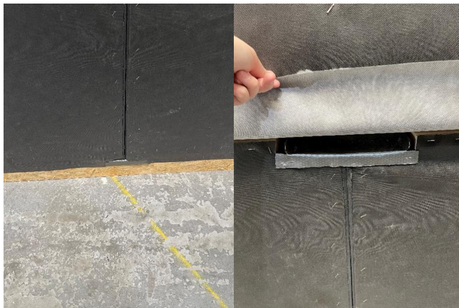
Figure 13: Water drip trays and waterproofing applied to the facade elements
