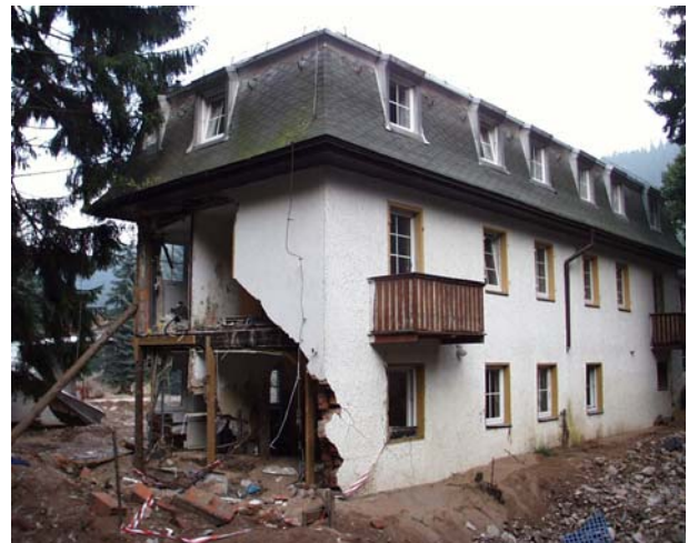
Fig. 1. Example of a close to collapse building with intact floor parts. Photo: Michael Markus.
