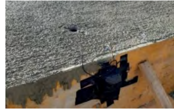
Figure 4. DS18B20 hardware module installed during concrete slab pouring
