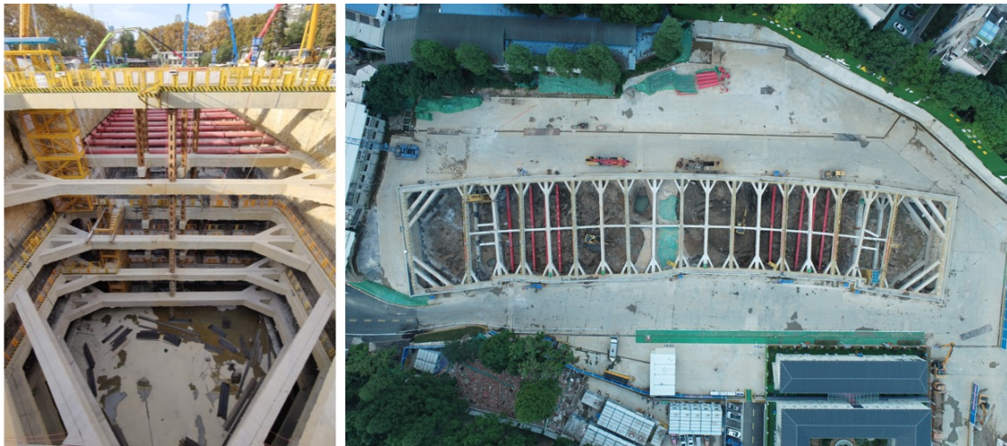
382 Figure 4. Example of deep pit foundation
