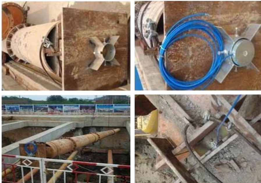
Figure 5. Examples of sensors installed in foundation pit
