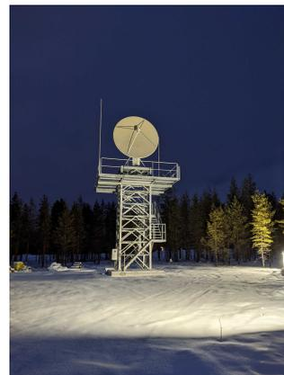
Figure 5: One of the two 3.7 m X/L band antennas in Sodankylä.
