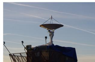
Figure 6: The X/L band antenna in Norrköping captured just after installation and without the Radome, 2011
