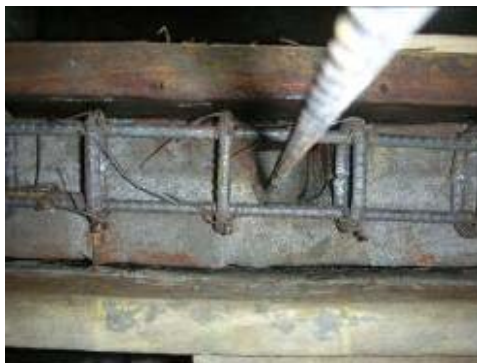
Fig. 5 Reinforcement Details @ junction
