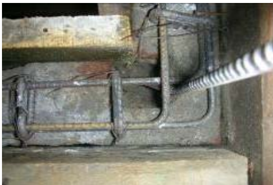
Fig. 6 Reinforcement Details @ corners
