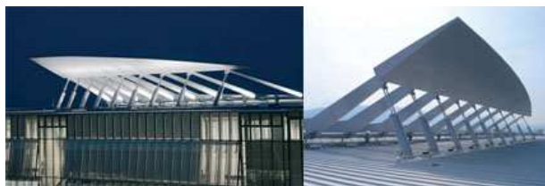
Fig. 4 The Transformable roof of the new Merck Serono Headquarter
